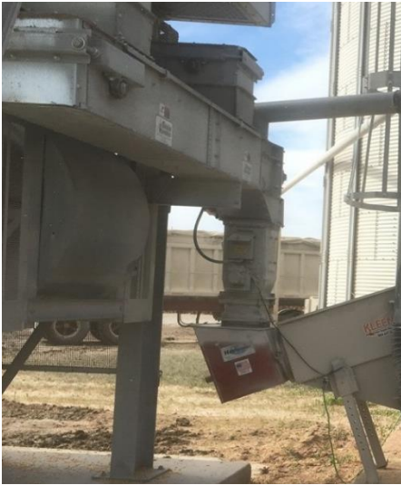
Figure 16 – In-line Chute installation
